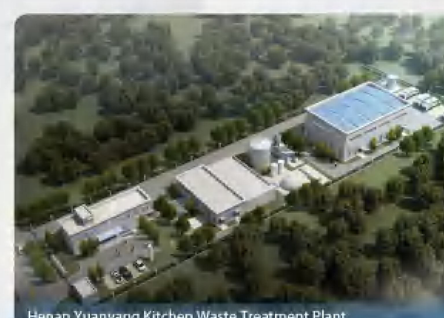
Henan Yuanyang Kitchen Waste Treatment Plant
