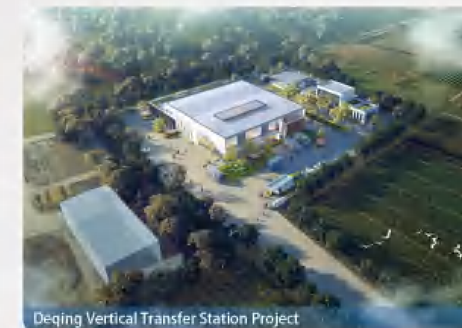
Deqing Vertical Transfer Station Project
