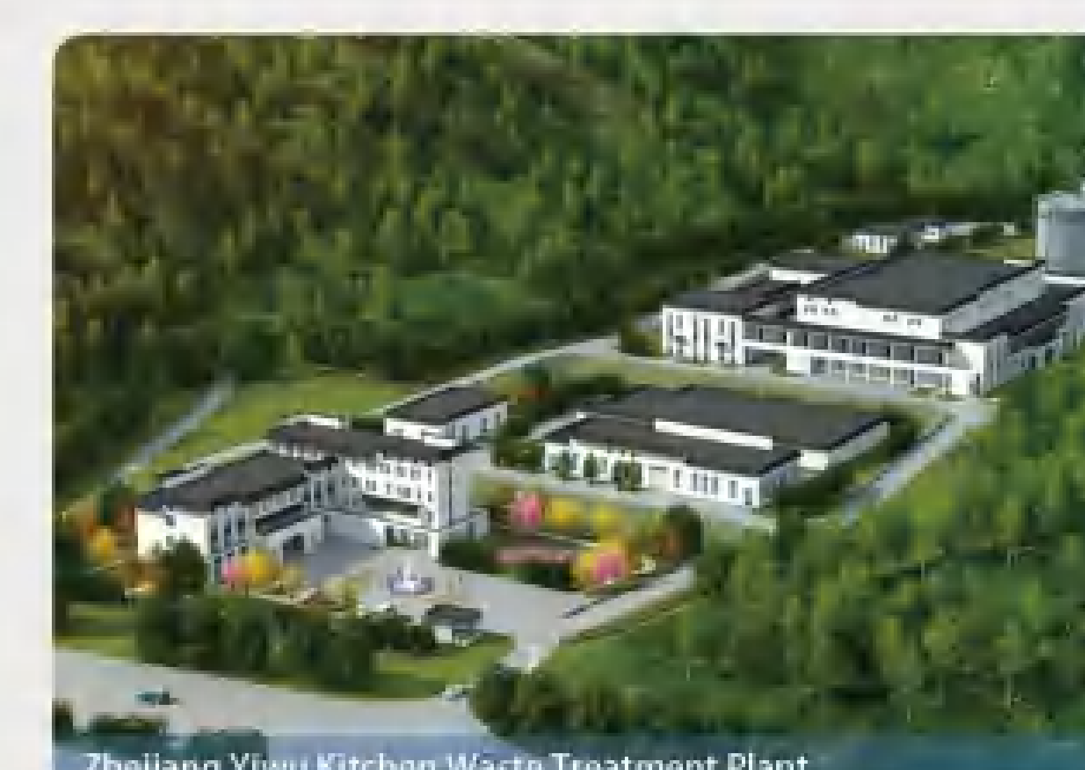
Zhejiang Yiwu Kitchen Waste Treatment Plant
